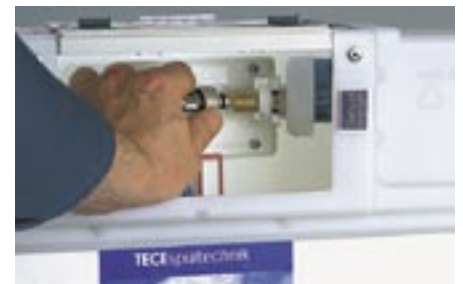
After the shell construction stage: The reinforced pipe is attached to the plug connection on the filling valve with no need for tools.
