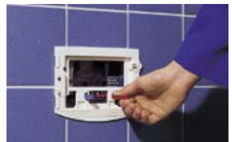
The push rods can be inserted quickly and accurately using the alignment marks.
